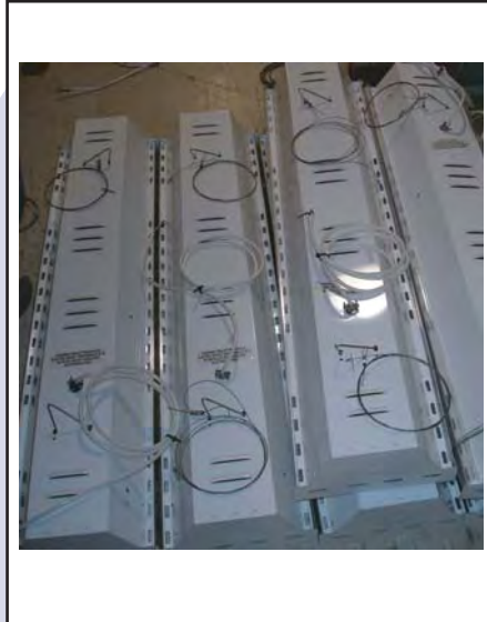
Pre-Installed hangers on fixtures
