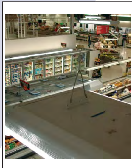
High Bay Fixture: Loop & V-clip
